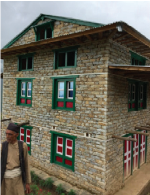
Figure 11. SMM house with shaped stones and low mortar-stone ratio
