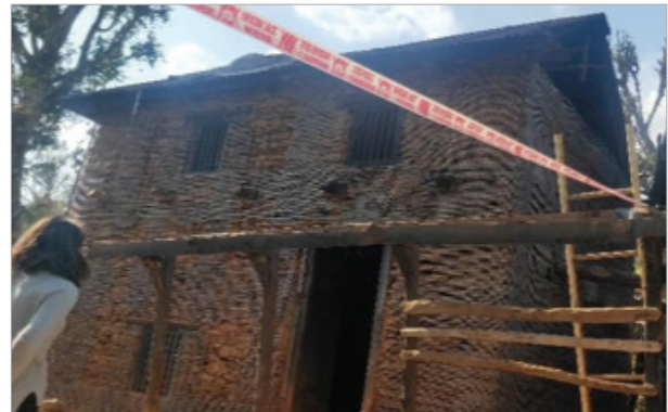
Figure 9. Splint and bandage retrofit of actual house
