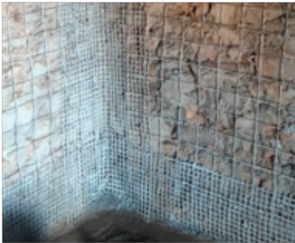
Figure 13. Application of GI wiremesh in Splint and Bandage retrofit
