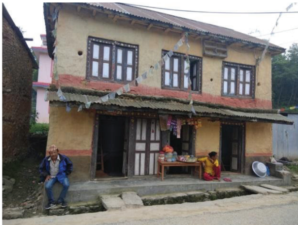
Figure 2. An SMM house with a store front in Kavre with large openings at the ground floor
