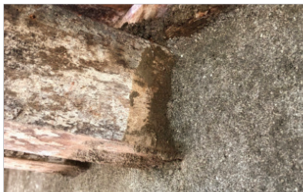
Figure 15. Timber member embedded in cement plastered SMM wall
