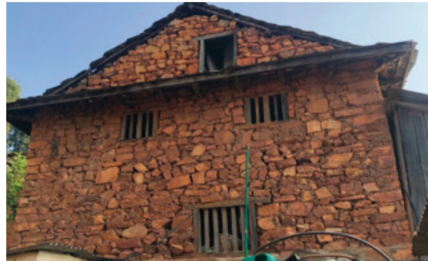
Figure 12. SMM house with angular stones and low mortar-stone ratio
