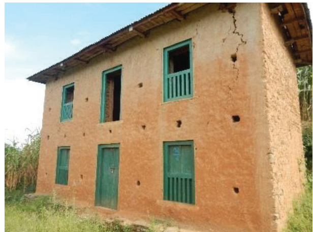
Figure 3. An SMM house without store front Sindhupalchowk
