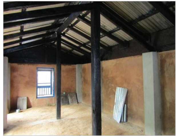
Figure 7. House retrofitted with Strong Back approach
